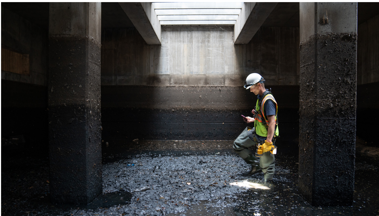
Figure 5. MWMO Monitoring and Instrumentation Specialist Brian Jastram inspects the Lowry Avenue Bridge's sand filter chamber on September 13, 2022.
