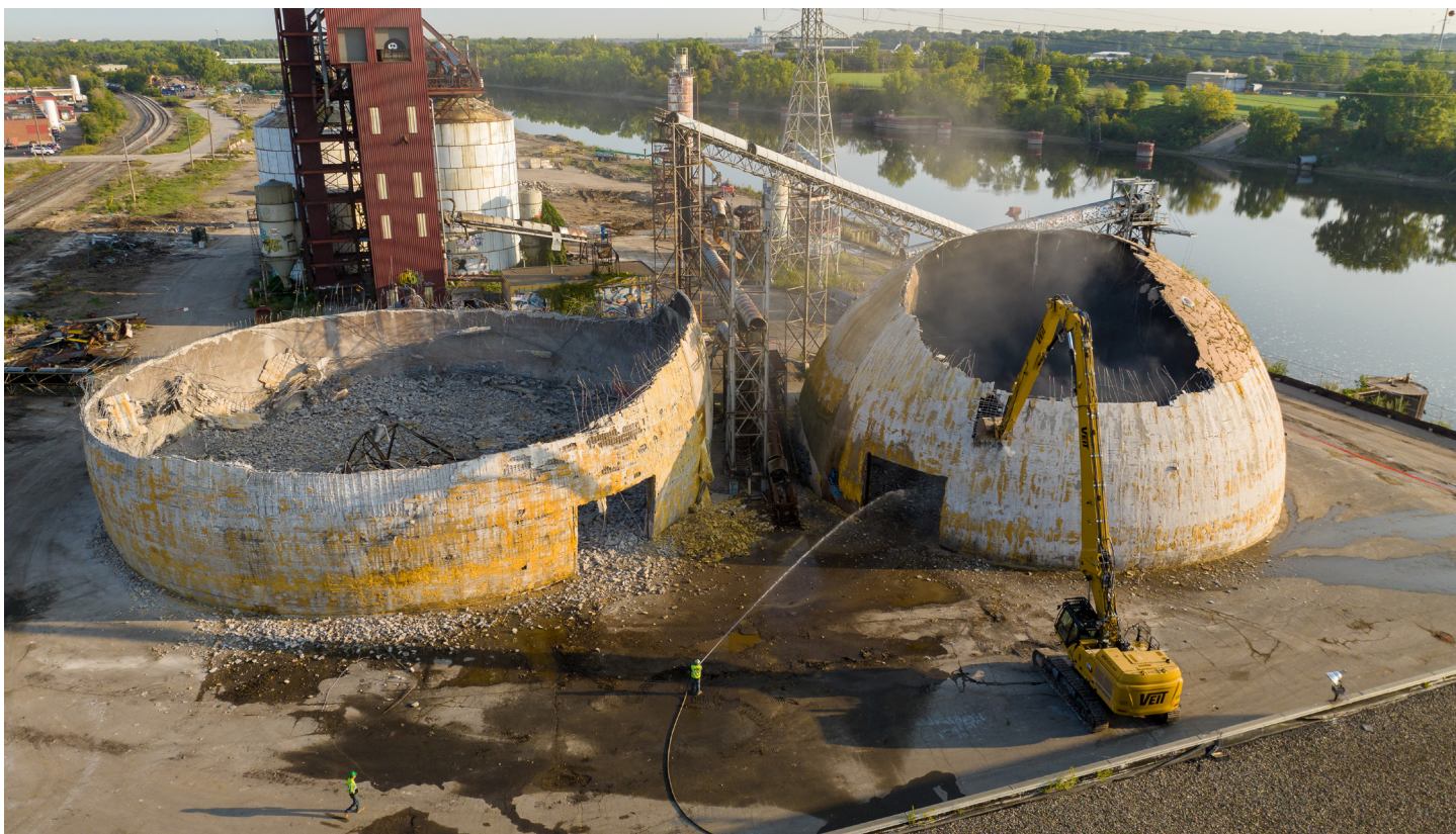
Figure 2. Workers use an excavator to demolish the dome-shaped silos at the Upper Harbor Terminal site in September 2022.
