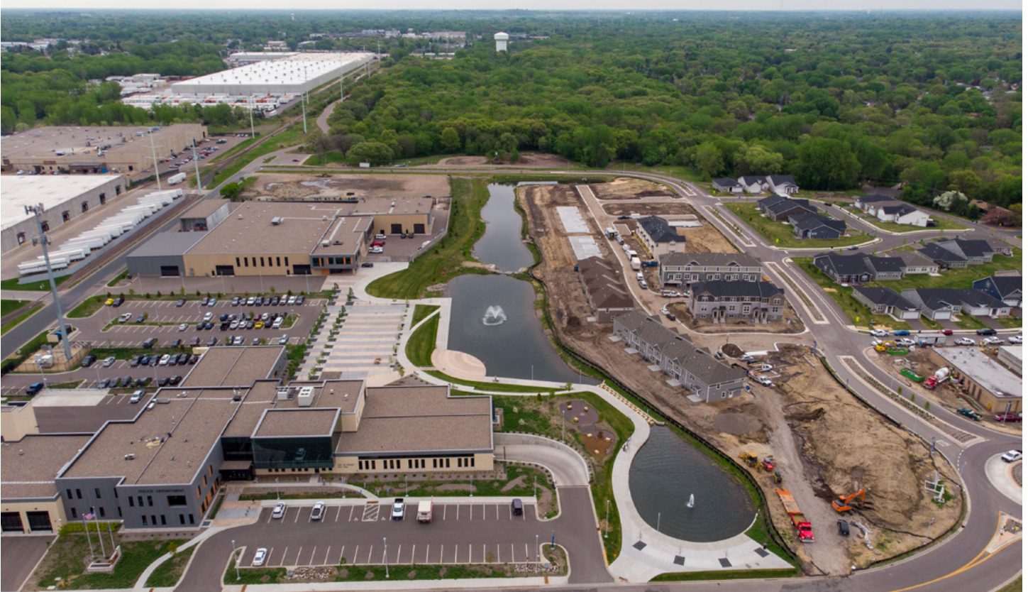
Figure 7. An aerial view of the City of Fridley's civic campus and its stormwater treatment train.
