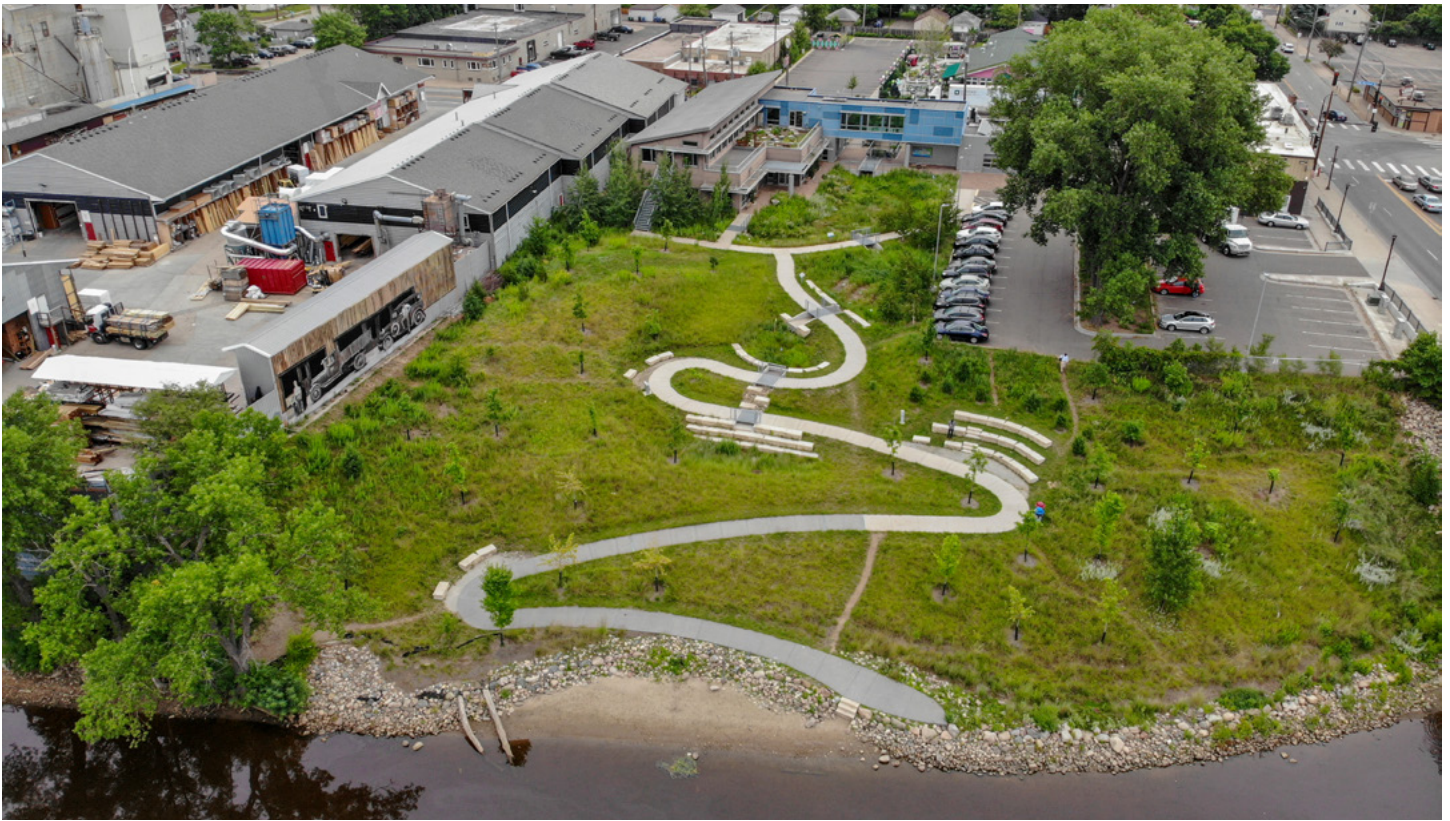
Figure 1. An aerial view of the MWMO's Stormwater Park and Learning Center in Northeast Minneapolis.
