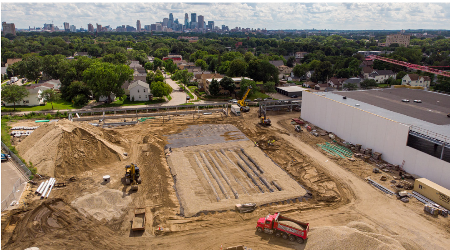
Figure 2. An aerial view of the underground stormwater infiltration gallery under construction at the East Side Storage and Maintenance Facility on August 15, 2019. The new City of Minneapolis public works facility includes a number of stormwater best management practices (BMPs).
