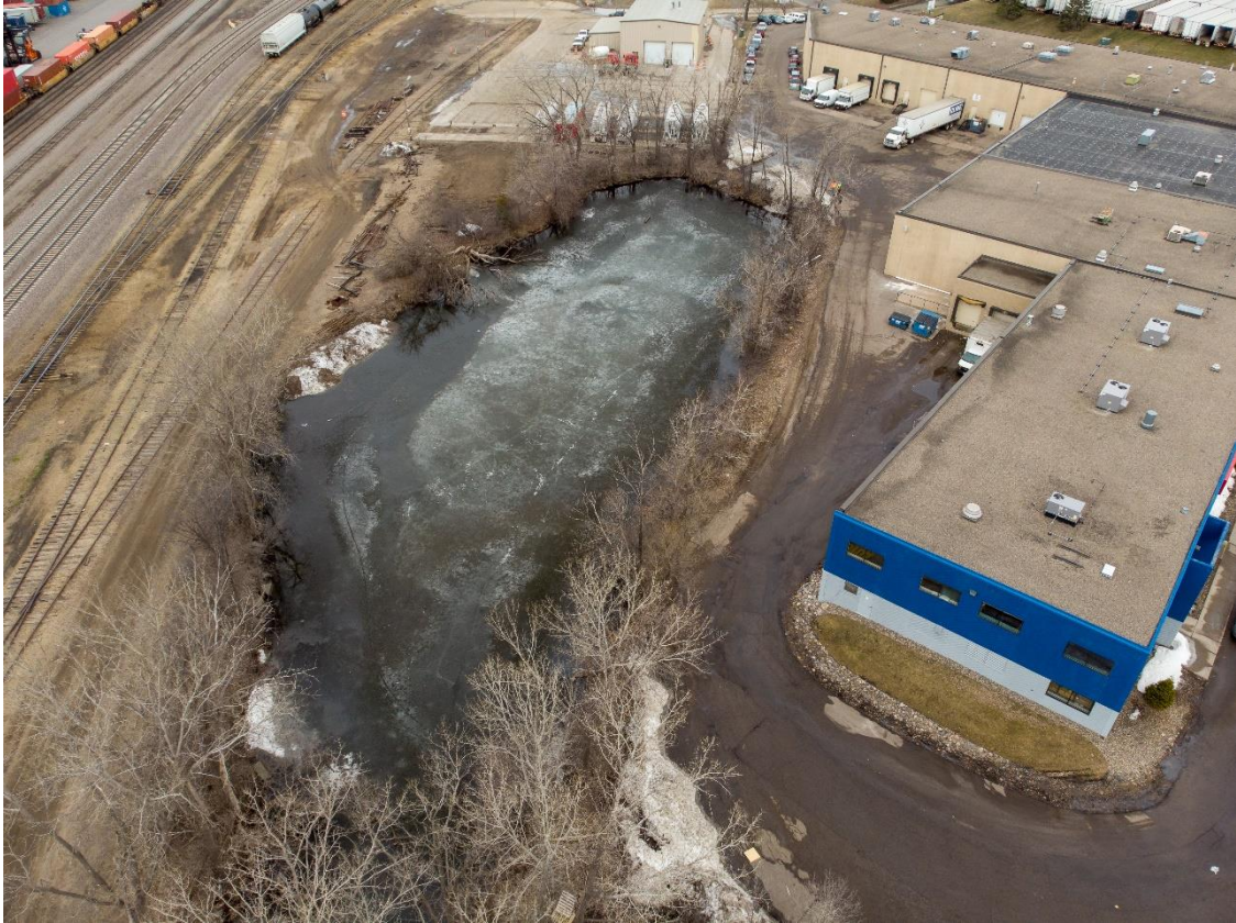
Figure 27. An aerial view of Kasota Pond West in March 2019.
