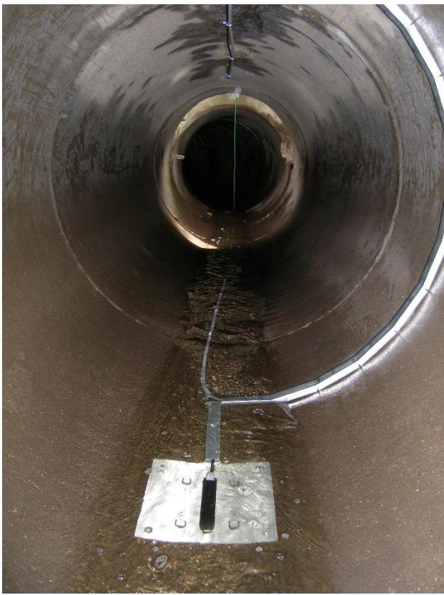
**Figure 5.** Typical area/velocity sensor (black rectangle) and cable configuration in a monitored stormwater tunnel
