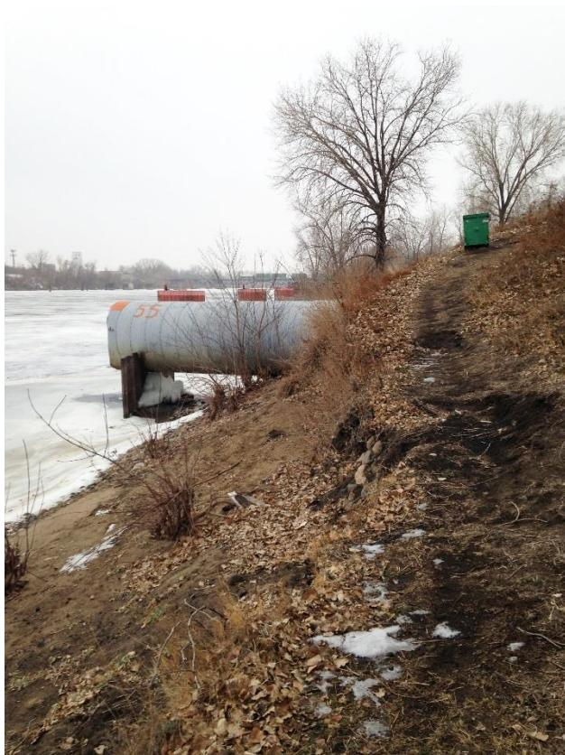
**Figure 10.** Outfall to the river for the 1NE pipeshed. Monitoring cabinet can be seen in the upper right corner (green box)
