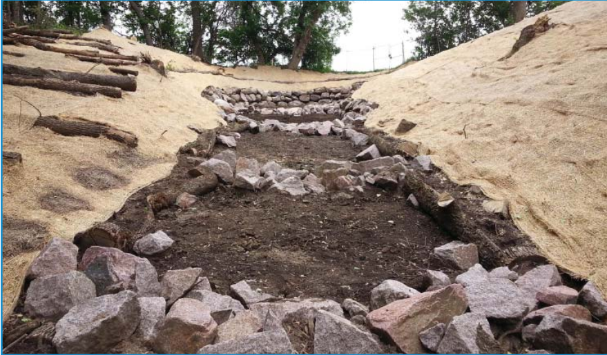
The ravine under construction, 2014
