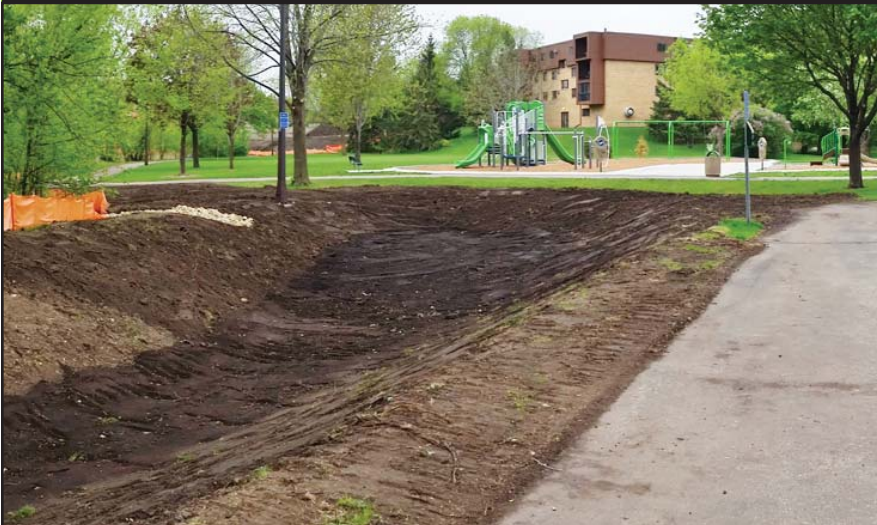
During construction, spring 2015
