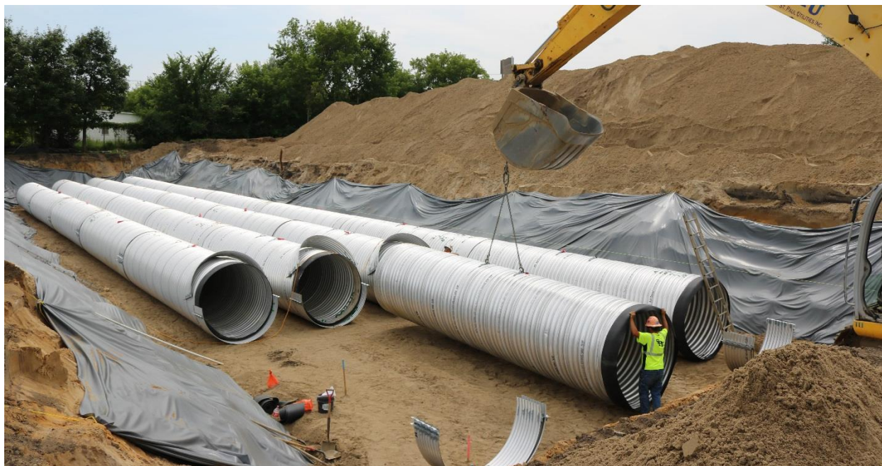
Figure 3. Workers install stormwater storage tanks next to the athletic field at Edison High School.
