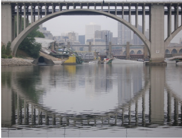
Figure 4. The Collapsed 35W Bridge
